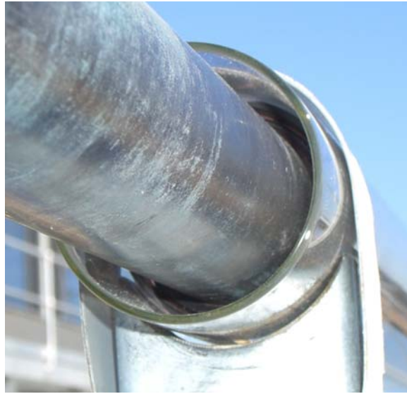
Figure 2.5 View of absorber tube inside glass tube
