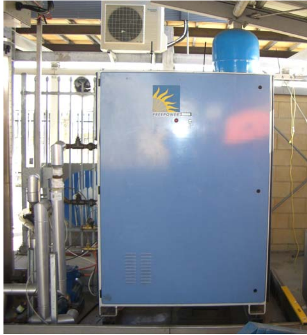
Figure 2.2. Freepower FP6 ORC unit at CSIRO
